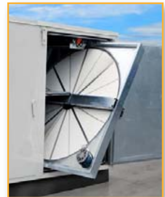
Rooftop unit with integrated Energy Recovery Wheel
