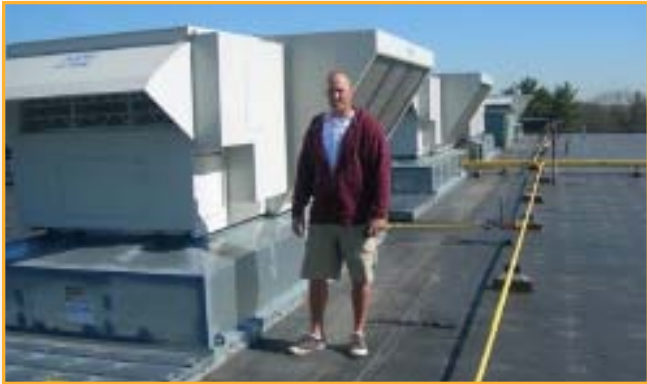
Custodian Tim Fournier comments there is no added maintenance for the energy recovery wheels.
